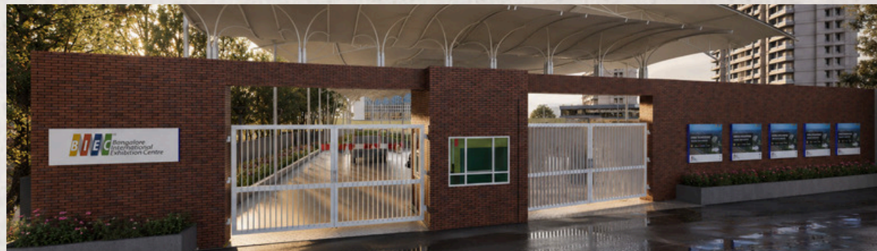
03 BIEC • CANOPIES, WASHROOM BLOCKS & INTERNAL RENOVATION
